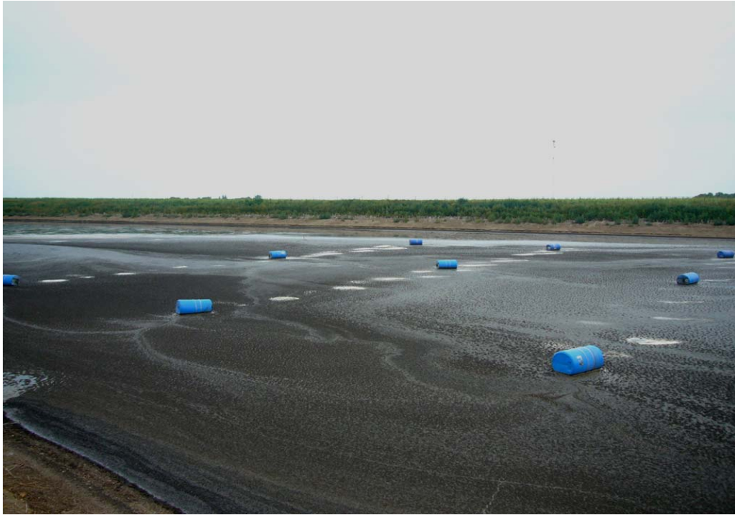
Figure 8. The actual placement of the aeration piping structure in a swine manure lagoon.
